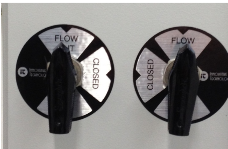
Figure 14 O 2 analyzer valves – Flow out and Flow in positions
